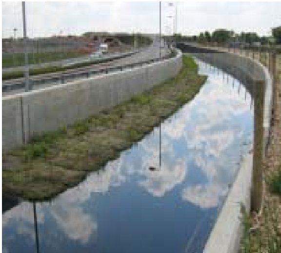
Site under construction
