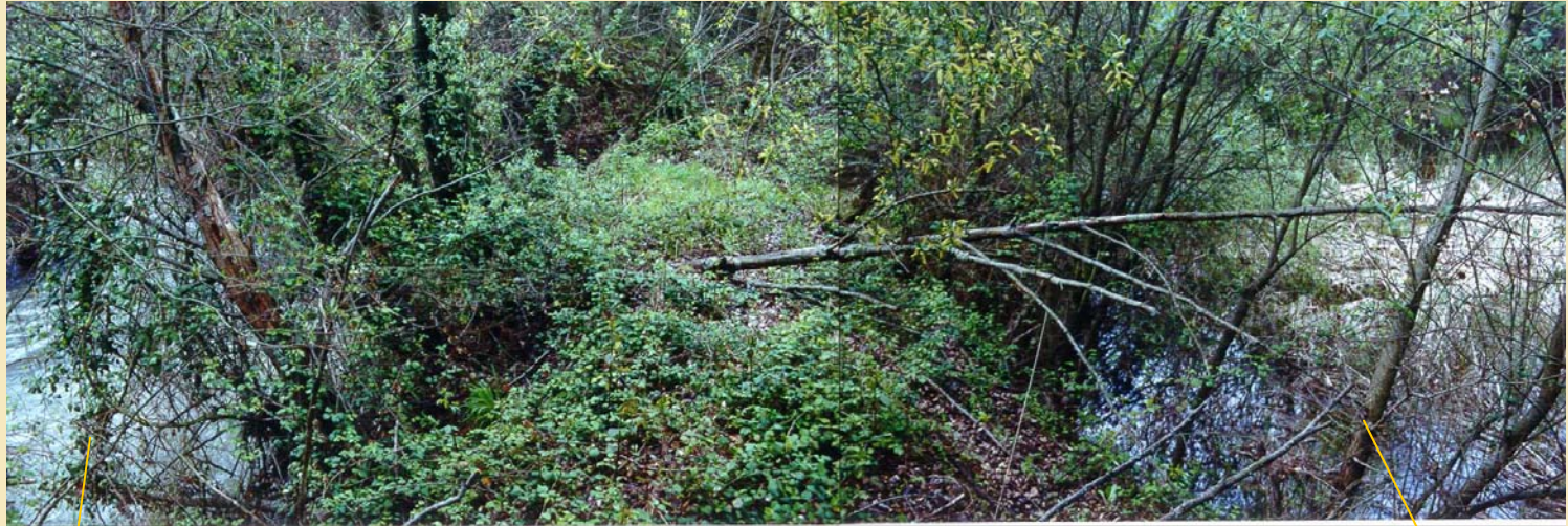
LEVEE (right bank)
